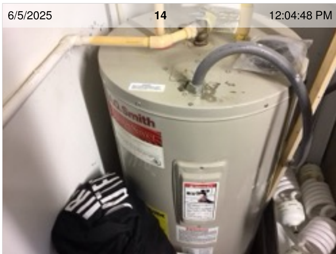
Electric Water Heater | A.O. Smith | Water heater (with expansion tank if present)
