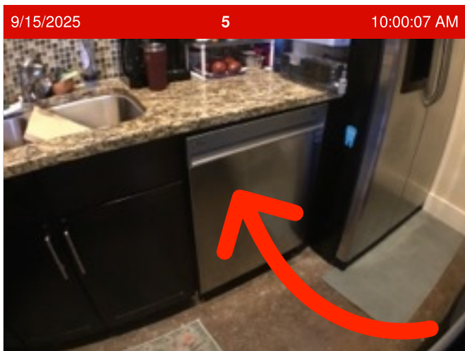
Dishwasher | LG | Exterior | Not fully mounted securely
