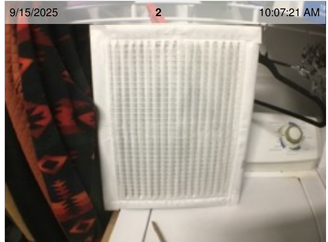
16 x 20 x 1 Air Filter | Front | TW 9-15-25
