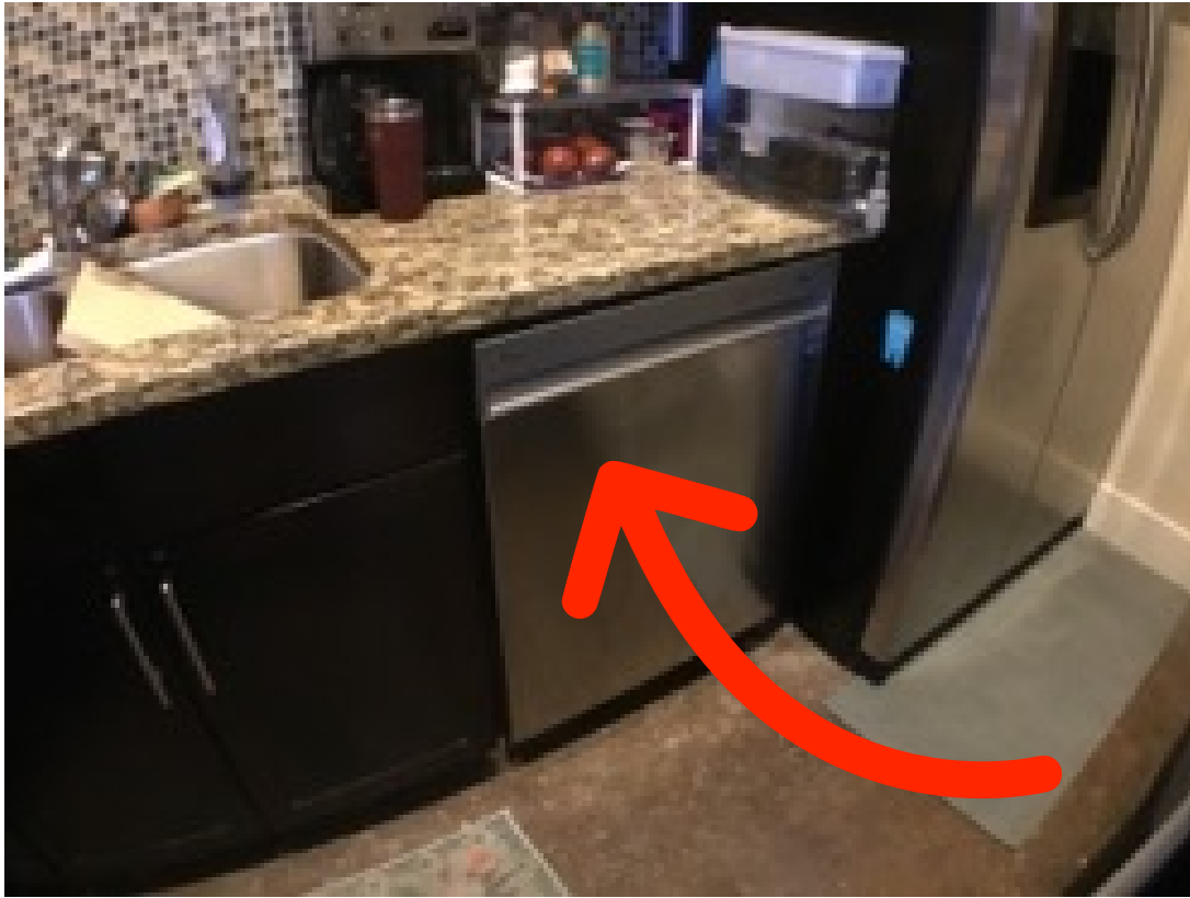
Kitchen Dishwasher Exterior Not fully mounted securely
