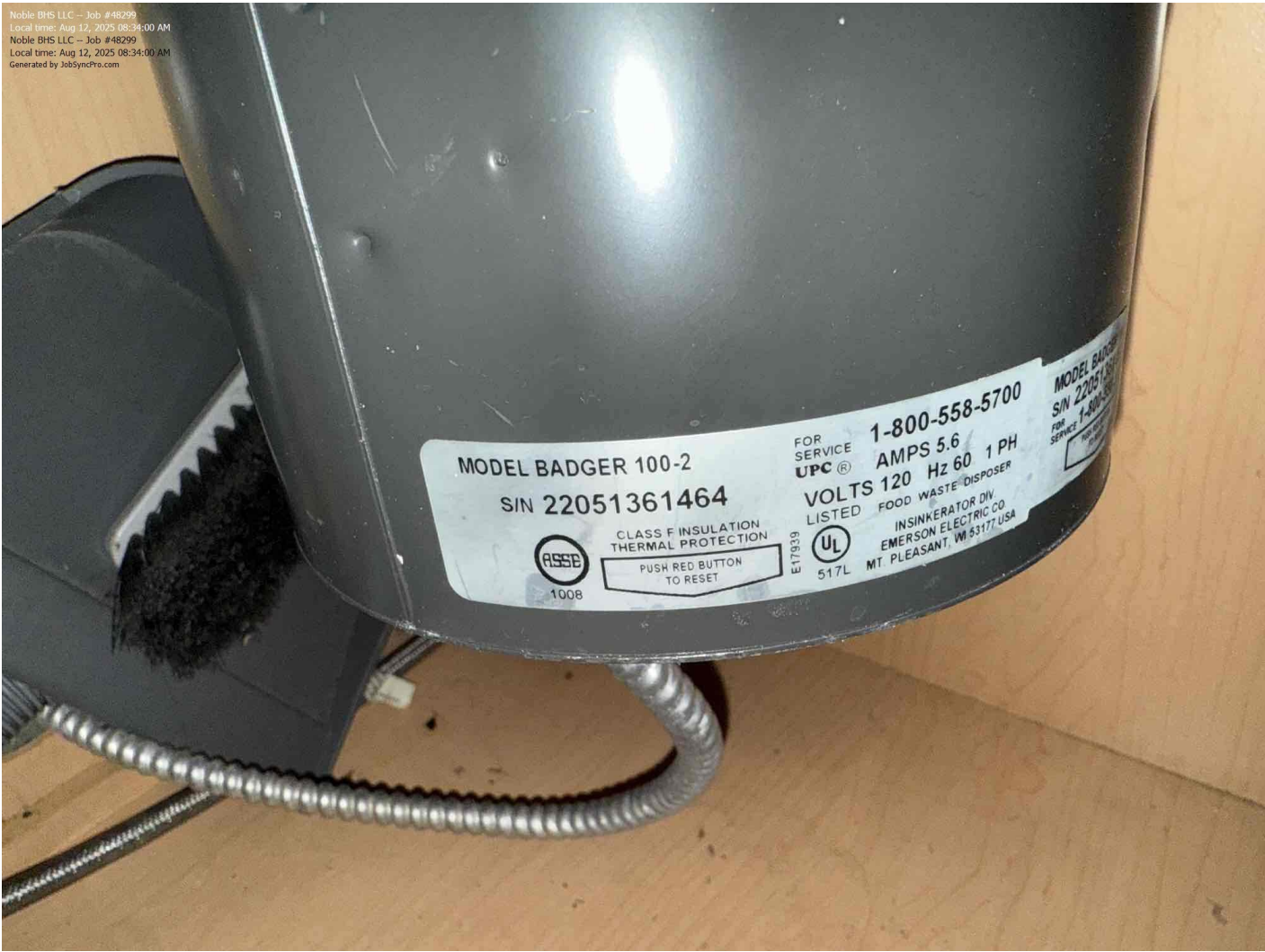
Motor was stuck I freed it
